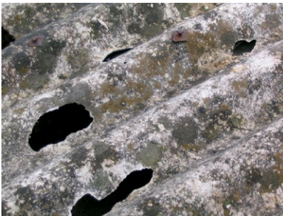
Asbestos fiber cement roof after the hailstorm
